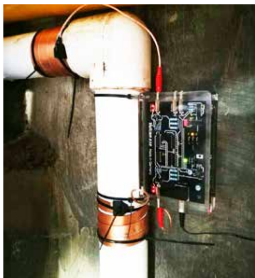
Vulcan S10安装在总出水管道上
