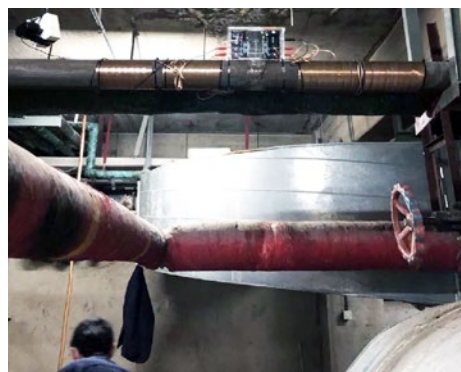
Vulcan S25安装在DN80铜管上
