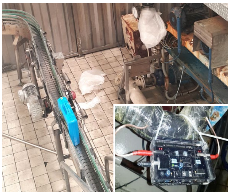
Vulcan 5000 is installed on the water inlet of the water recycling room.
