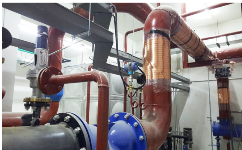
Vulcan S350 was installed in the heating system in the high zone of the heat exchange station.
