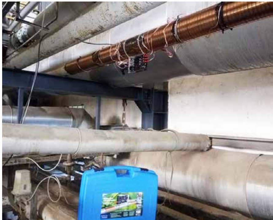
Vulcan S150 was installed on the main water pipe.
